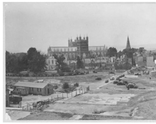
Rubble cleared, Cathedral
